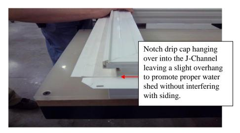
13.) Apply 4" tape over the drip cap at the mull location closing the backside of the drip cap and 1/2" nailfin gap. Also apply tape over any color matched silicone to provide a finished look.
